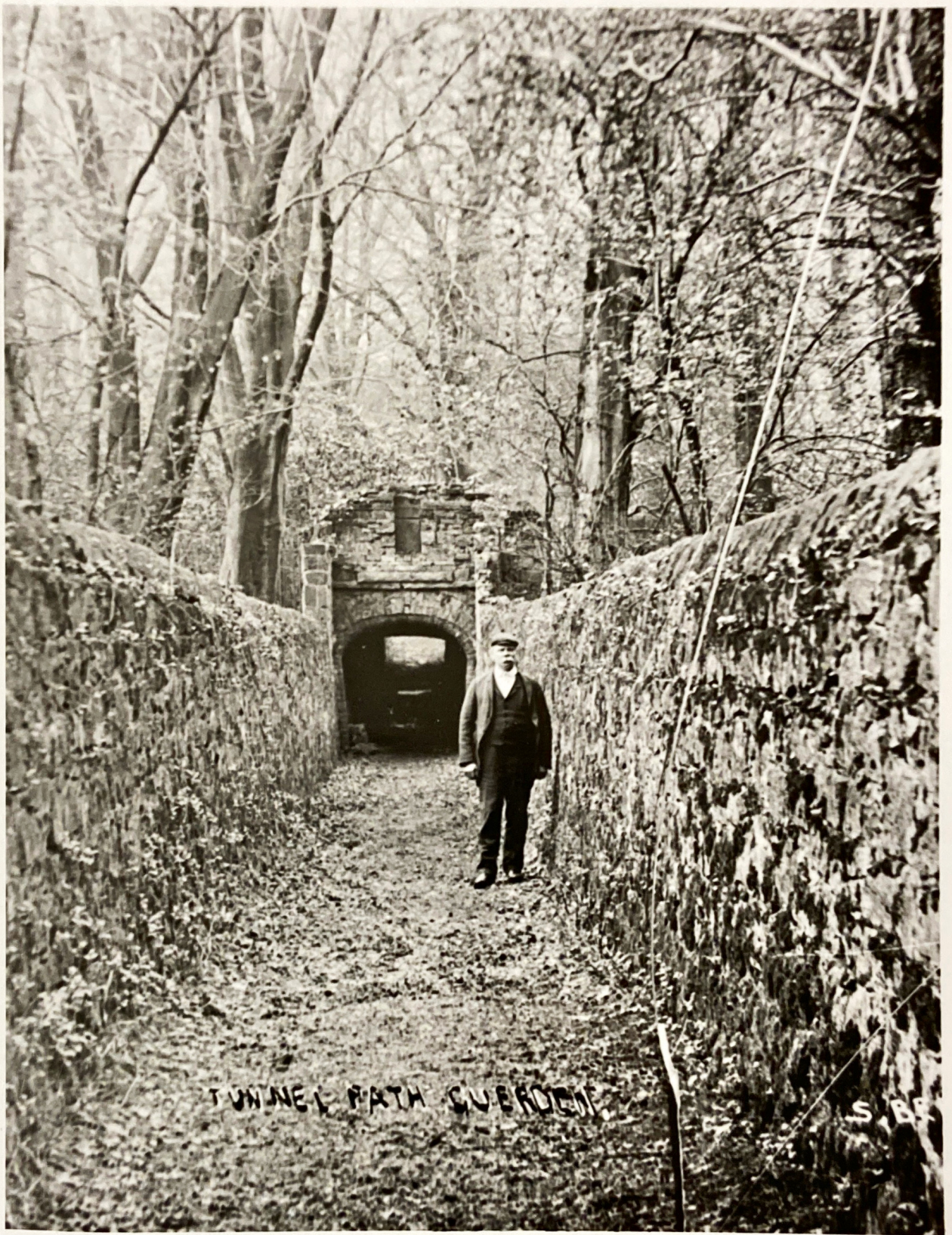
Tunnel path to conceal staff as they went about their business -from owner, Cuerden Hall. It became a public footpath
