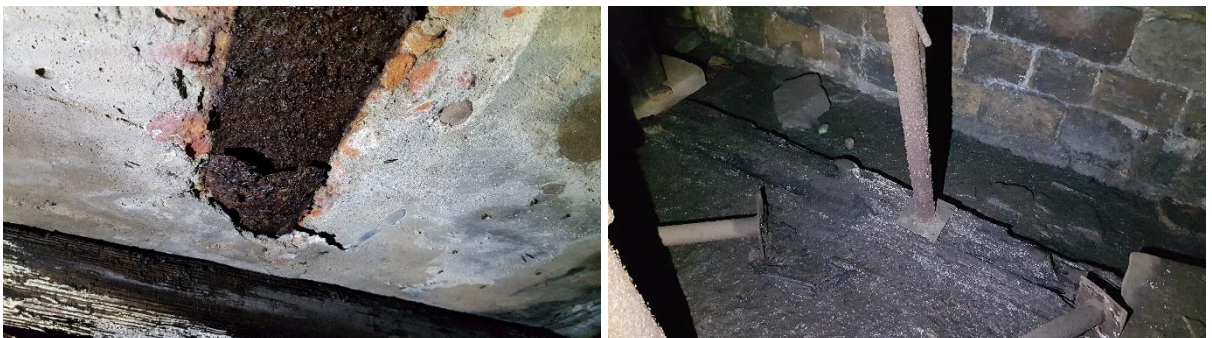
Figure 5: Concrete spalled and joists corroded (left), acrow props are corroding and the timber beams they were bearing on are decayed (right).
