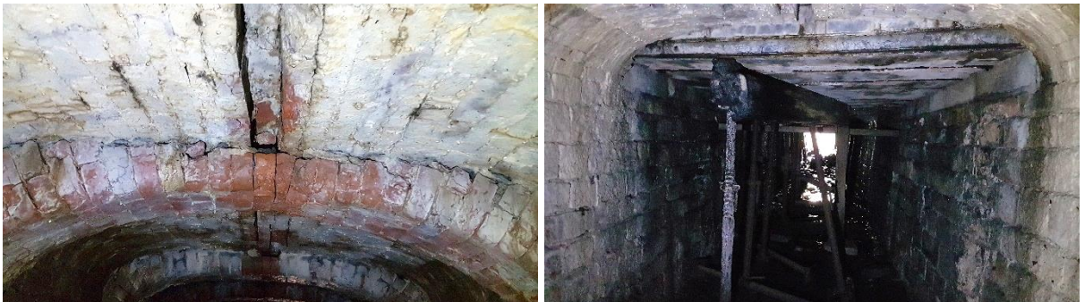
Figure 4: Arches unbonded and thinner at crown as if cut to fit deformed shape (left), and filler joist below road (right).
