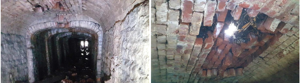
Figure 3: Deformed masonry barrel vault (left), and collapsed sections of vault with loose masonry units (right).
